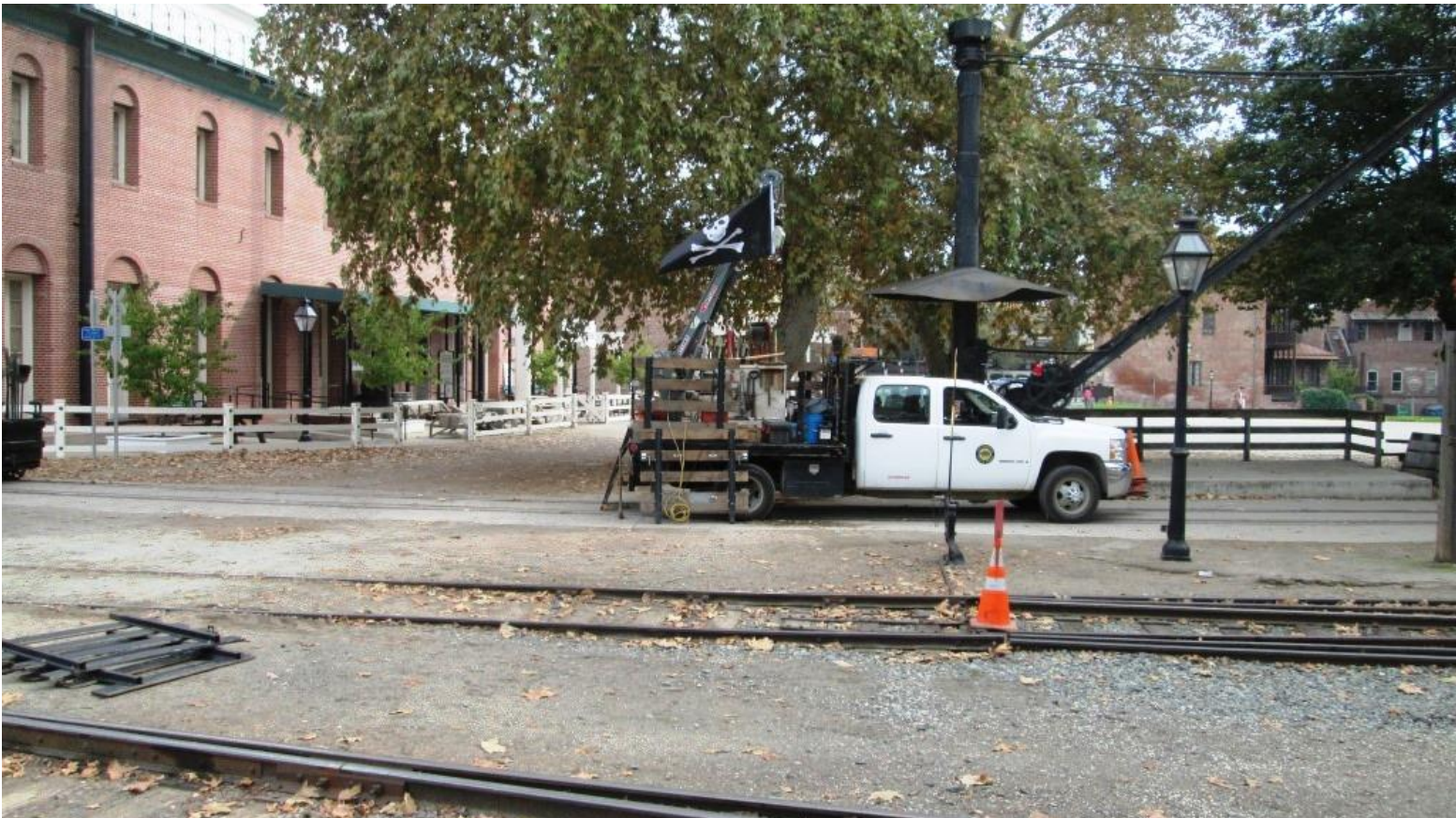
"Ahoy, mateys!" The Jolly Roger flies from the crane-mast of the MOW Team's trusty Chevy Truck
