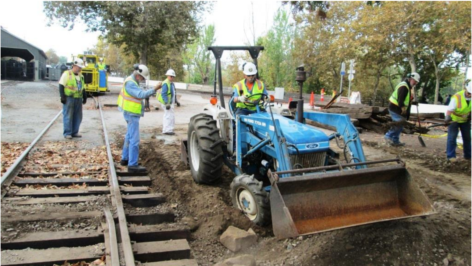
Joe grades the area to the west of the track with the blue-tractor
