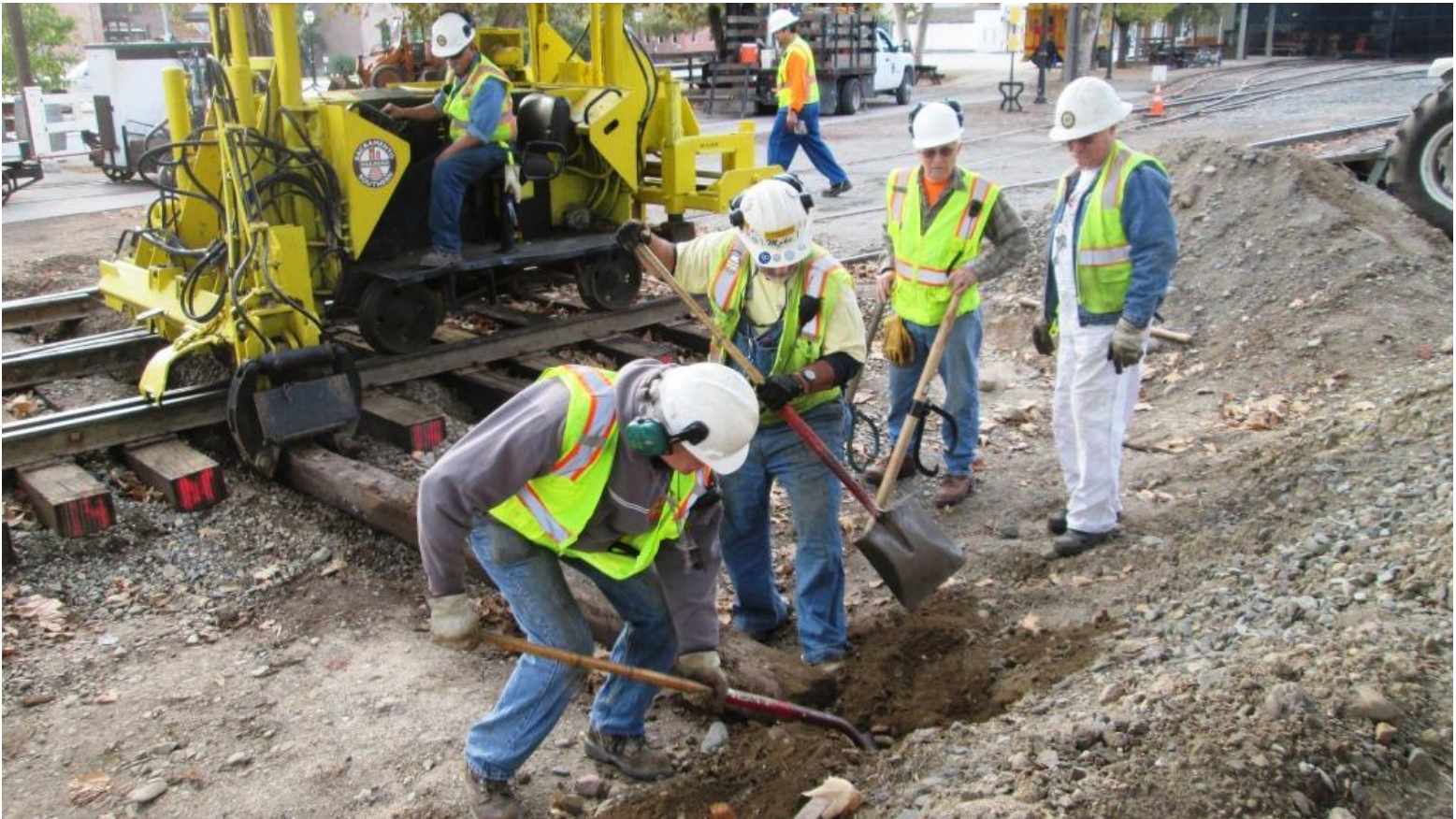
Steve and Mike F. dig a trench to give the tie a little more room to slide out
