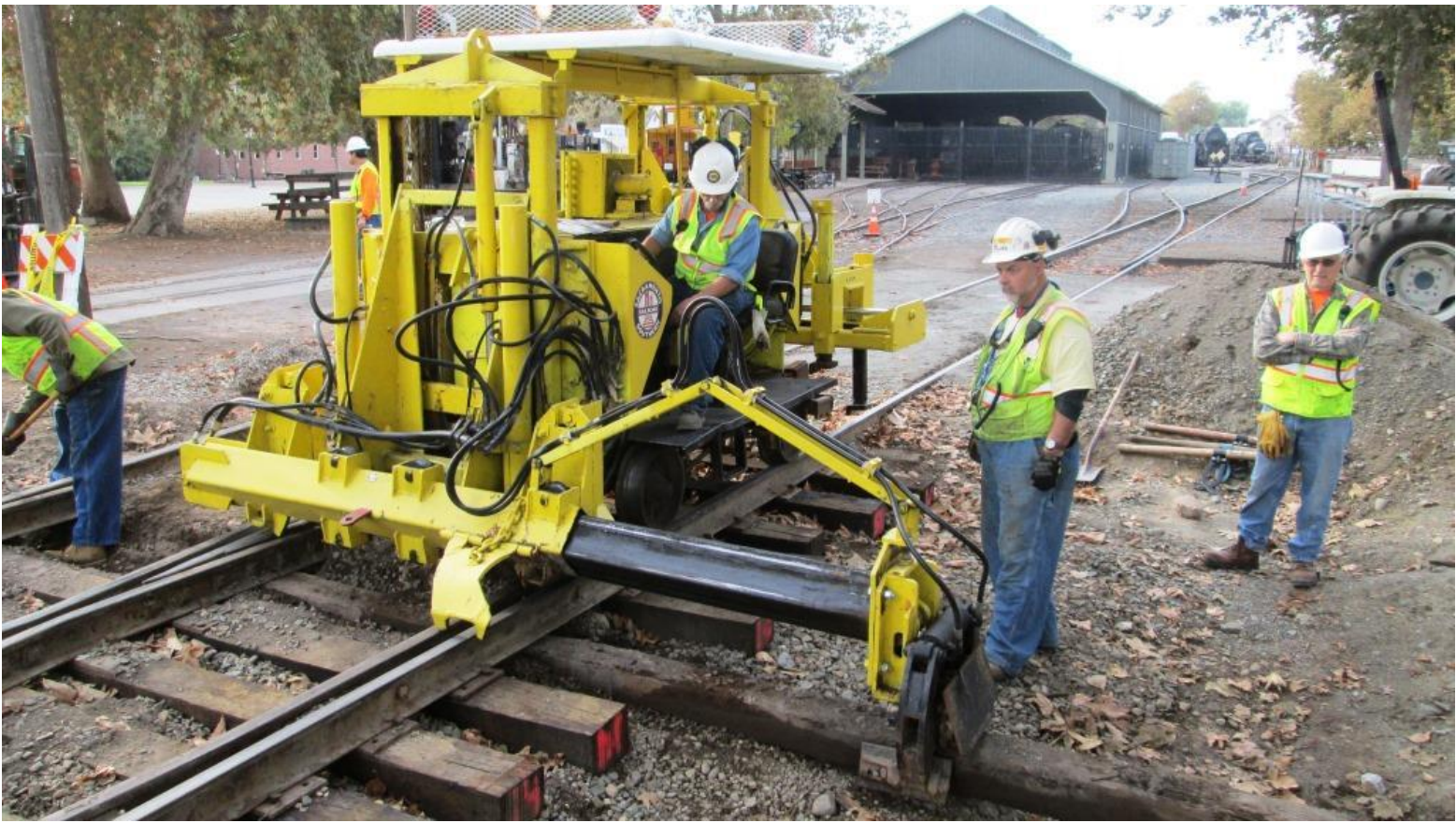
Joe uses the Jackson 125 tie-exchanger to remove that last tie slated for replacement at the Switch 1 Turnout
