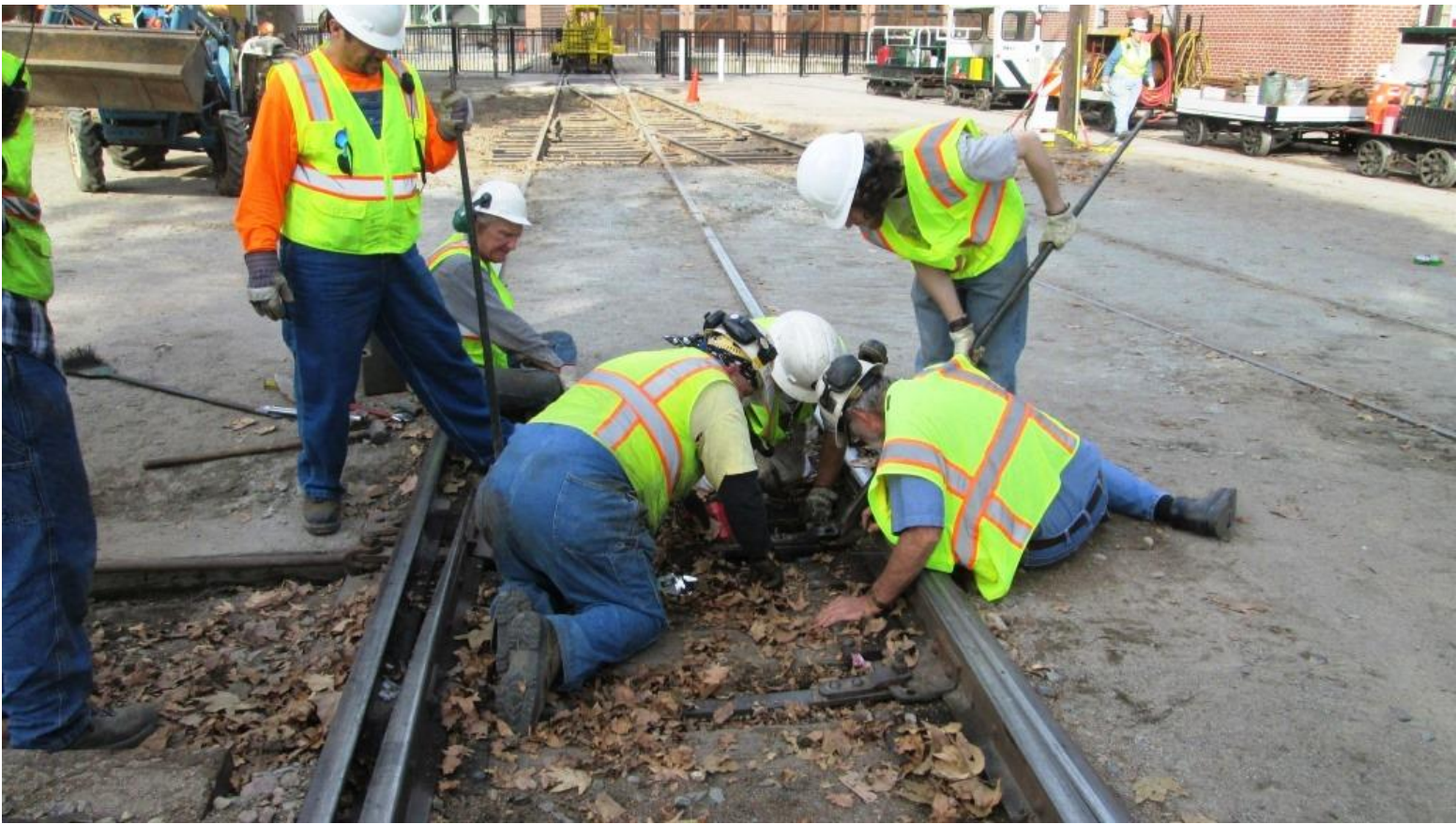
Matt uses a lining bar to lever-up a bolt from underneath the transit-clip and Mike F., Mike H., and Alan line up all the bolt-holes
