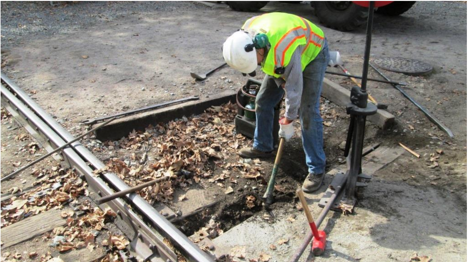
Steve digs out the switch-rod side of the head-block to make room for the new switch-rod
