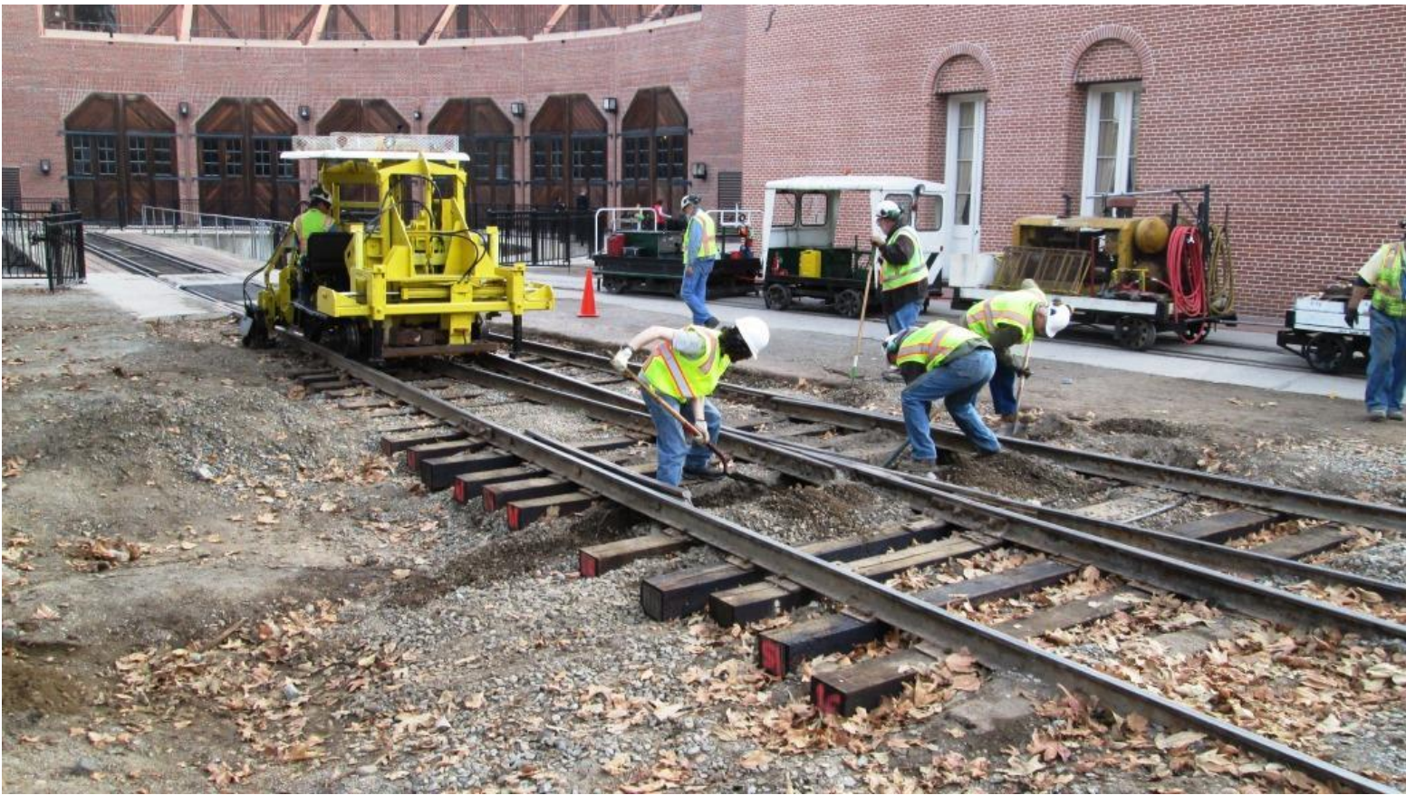
With the tie now removed, Matt, Steve, Clem, and Frank dig out the tie-crib
