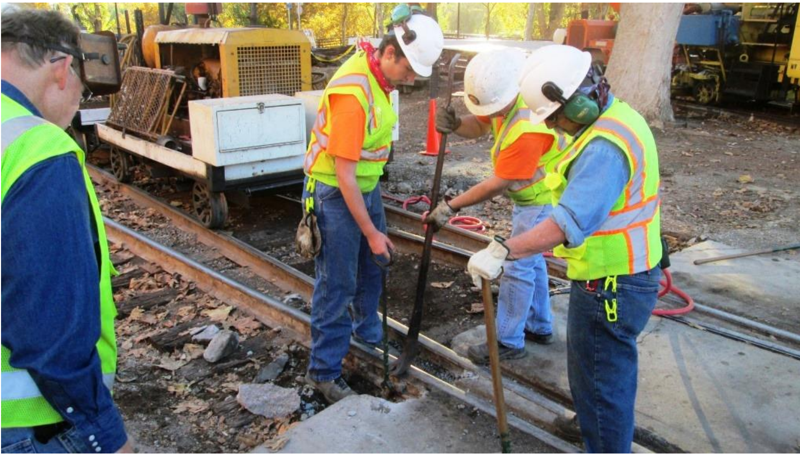
Weston employs the road-master tool on the head of the spike as Mike H. pulls it using the claw-bar
