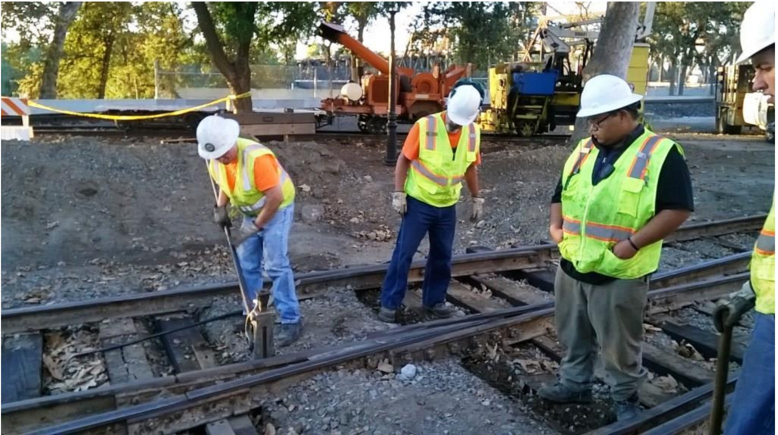
Mike H. uses a track-jack to relieve downward pressure on the tie-plates for easier removal
