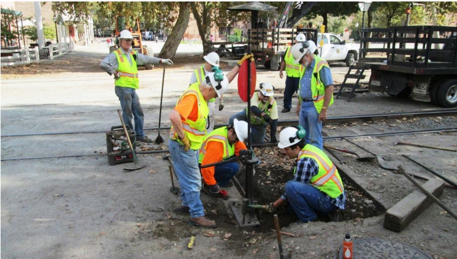
Weston and Jose set spikes at the base of the switch-stand
