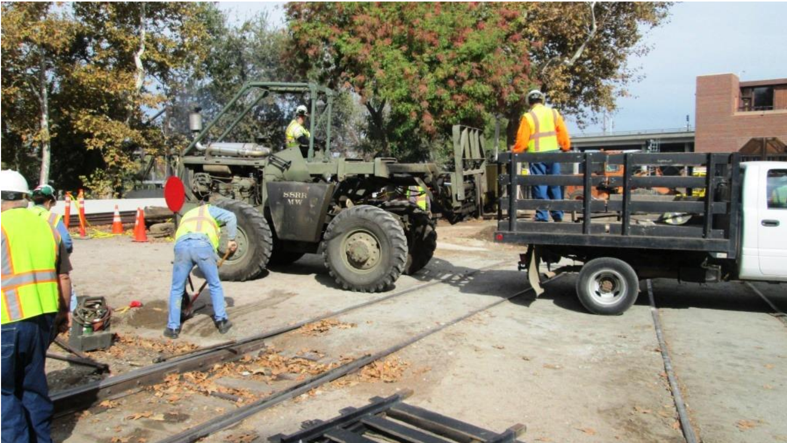
Following the "incident", Mike F. on Big Green loads the unfortunate switch-stand into the bed of Truck 14
