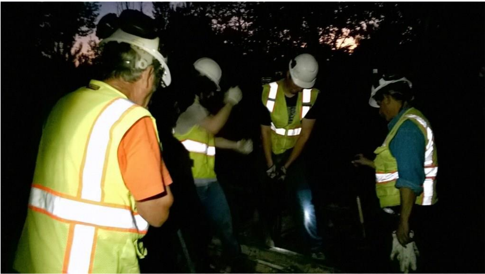
"Rage against the dying of the light..." Weston uses the road-master tool so that Matt, with the claw-bar can pull the spike
