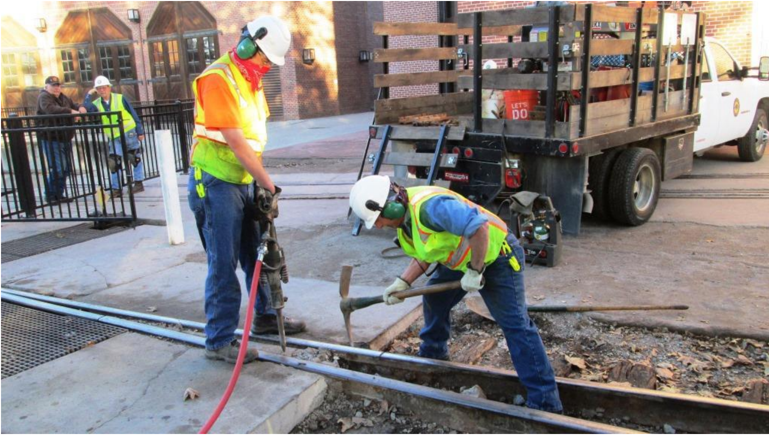
Weston and Joe remove a few bits of concrete from around the joint the Team was fixing
