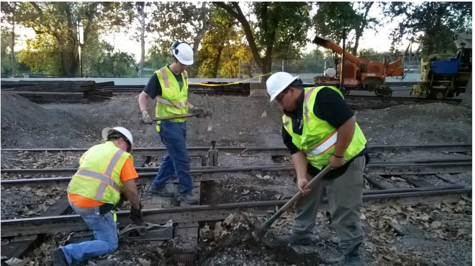
Mike H., Weston, and Anthony place jacks horizontally to shove a catawampus tie wampus...
