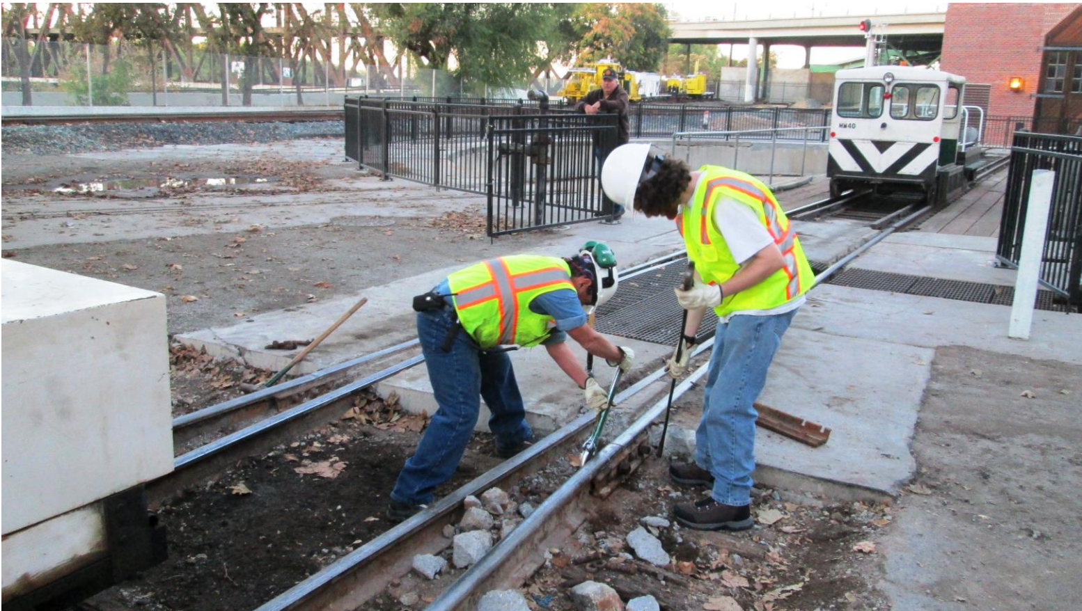
Joe and Matt tighten-down the new bolts
