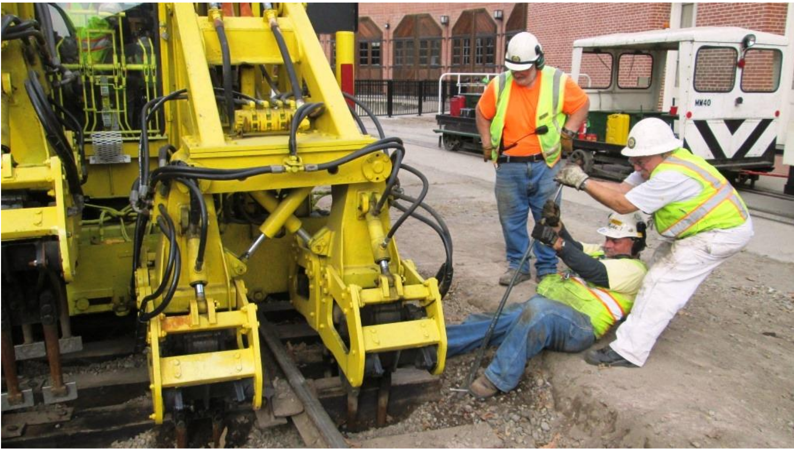
Meanwhile, back at the Switch 1 Turnout, Mike F. and Mike H. struggle to nip-up a switch-tie as Steve in the tamper tamps it up
