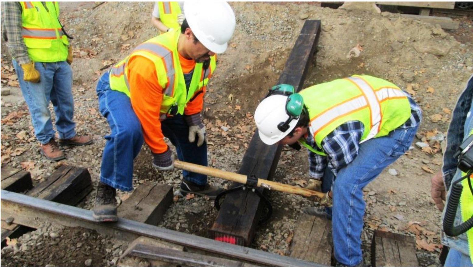
Jose and Weston position the tie for insertion
