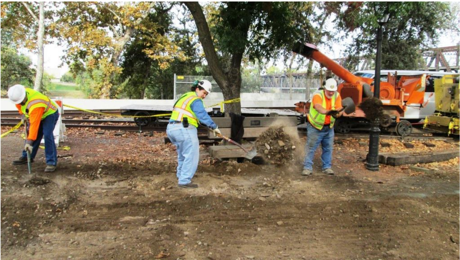
Jose, Heather, and Frank shovel more soil into the area being graded
