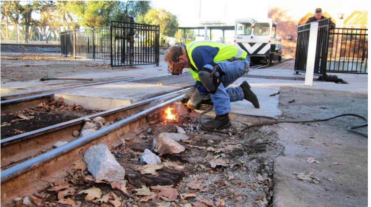
Cliff cuts a corroded bolt by focusing the heat of a volcano with his cutting torch
