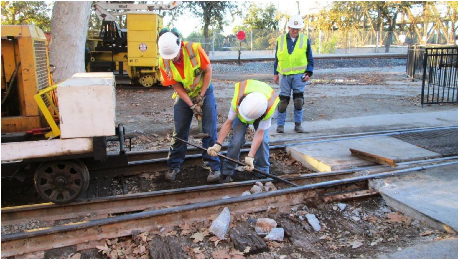
Weston and Matt use a lining bar to pry the joint-bar off the track
