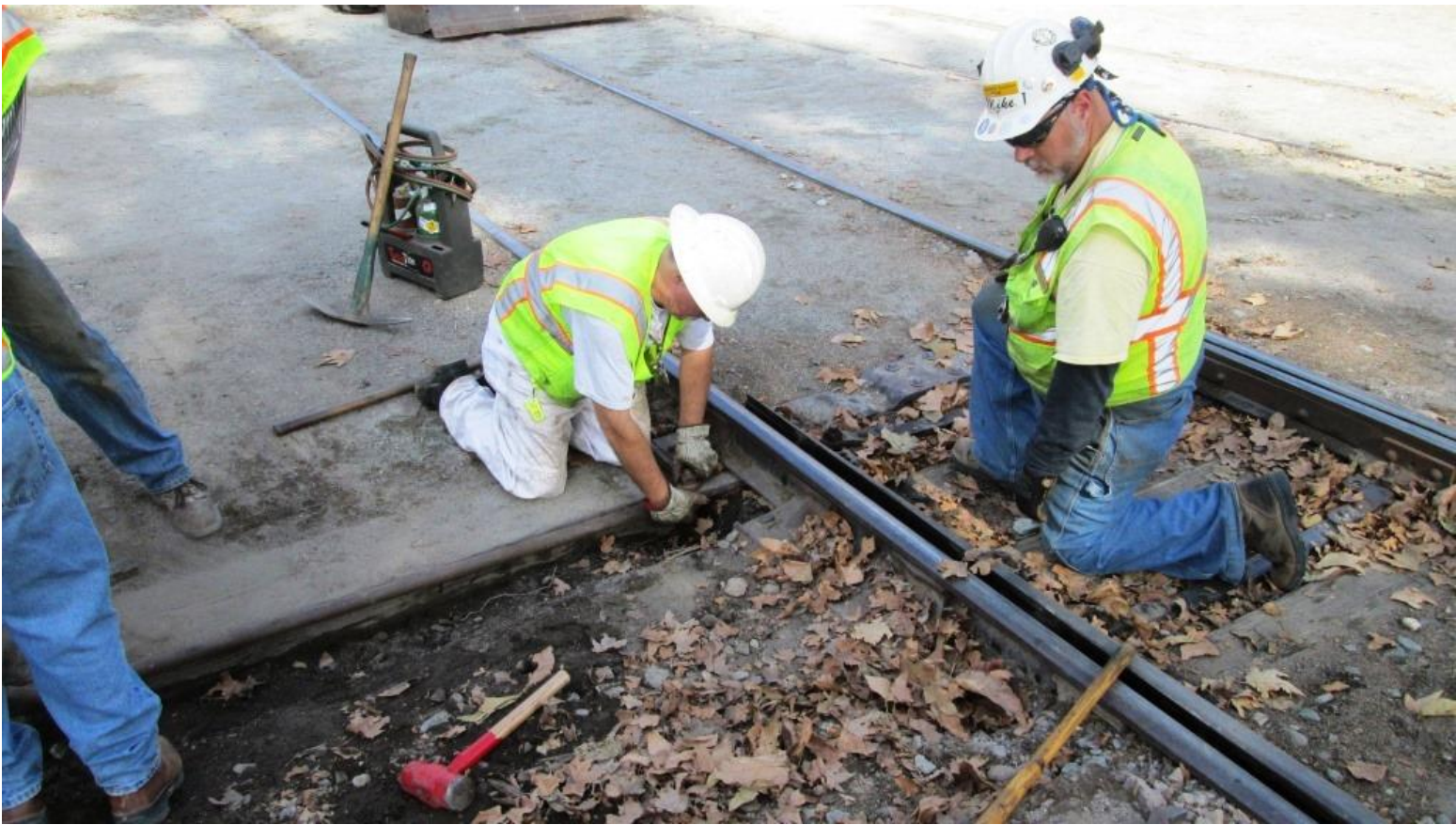
Mike H. and Mike F. work to connect the new switch-rod to the connecting-rod under the switch-points
