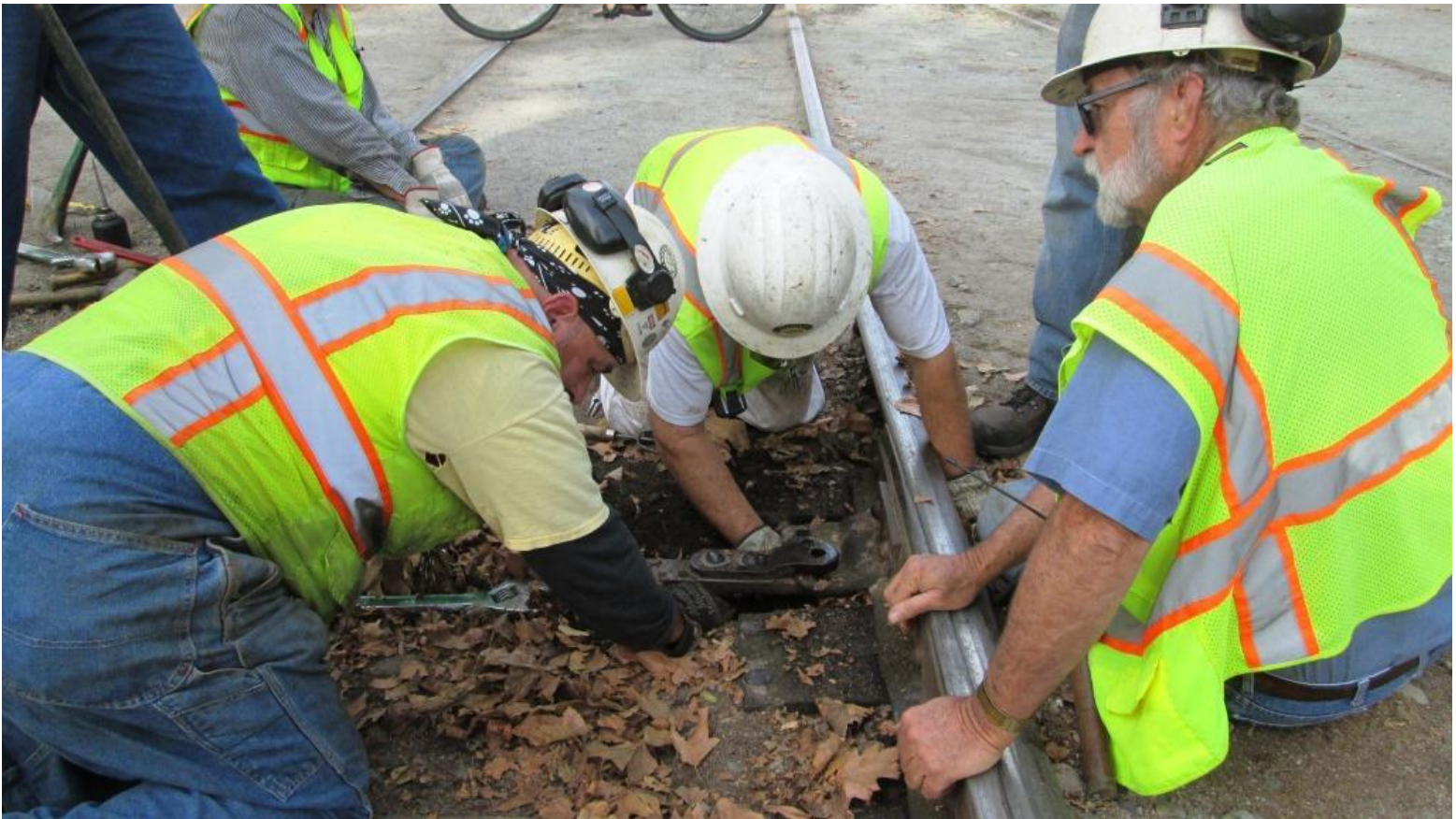
Now to adjust the switch to the new stand: Mike F., Mike H., and Alan adjust the position of the connecting-rod in relation to the transit clip
