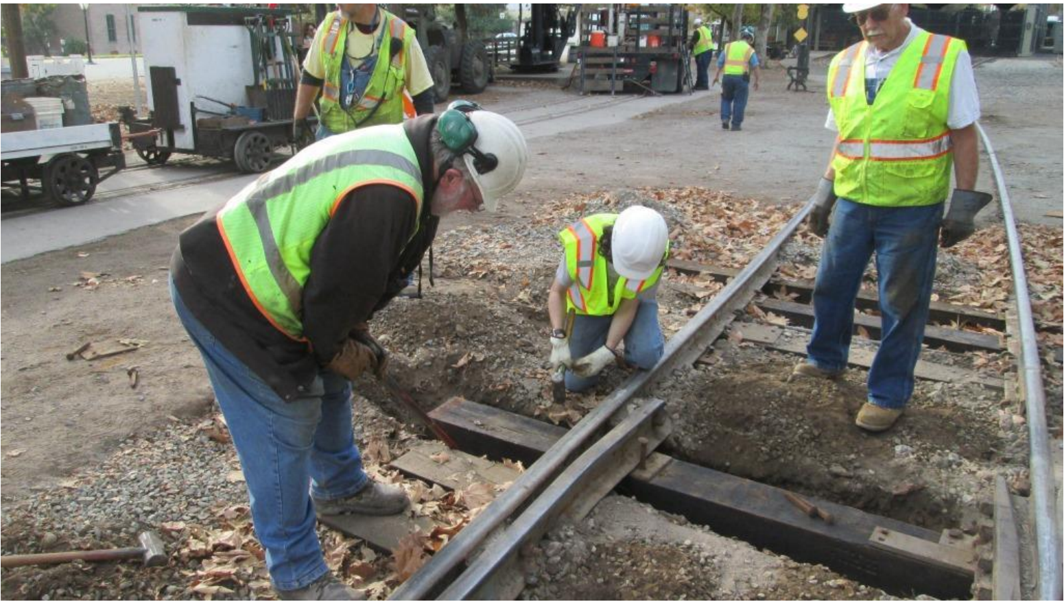
Frank nips-up the new tie as Matt sets spikes
