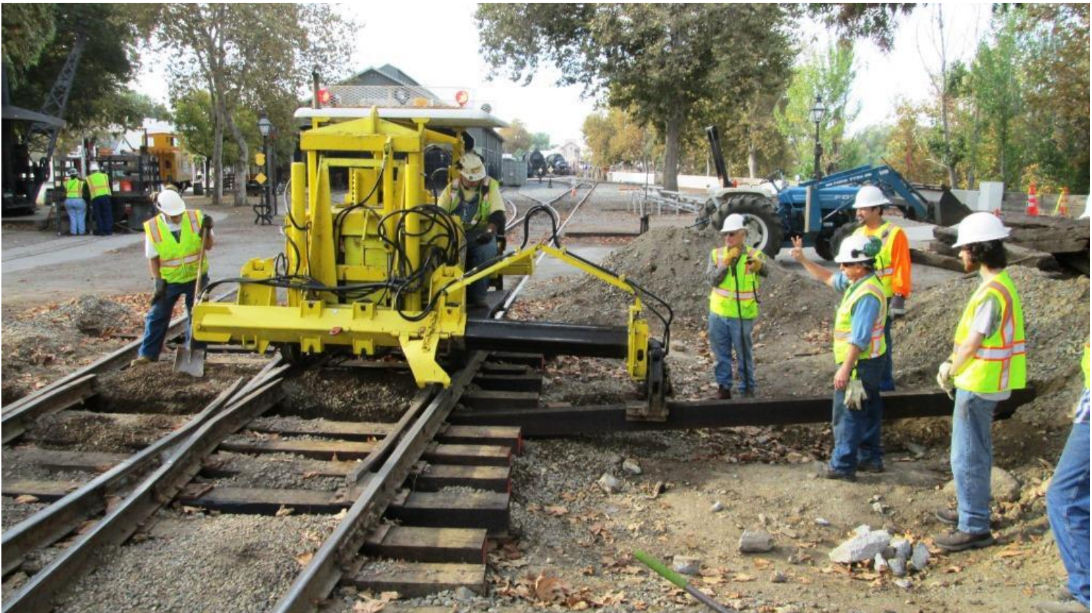
With Joe as guide, Mike F. tries his hand at inserting a tie
