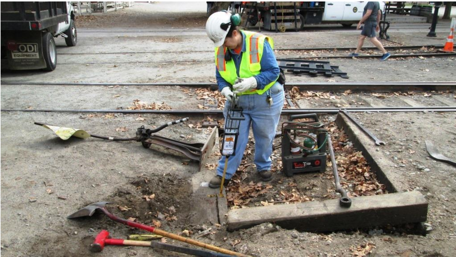
Heather injects epoxy-goo into the shattered end of the head-block
