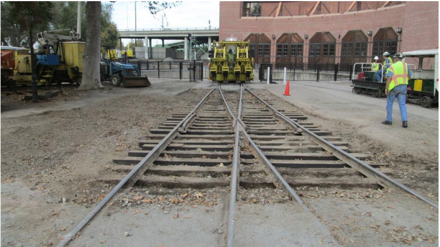
It's looking pretty good: cleaned-up and ready for rock, the Switch 1 Turnout looks solid!
